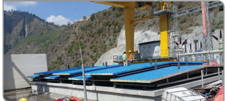
Gulpur Hydropower Project | Roofing System 4,000 Sft
