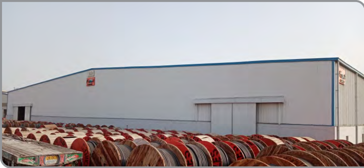
Fast Cable | Warehouse 110,000 Sft
