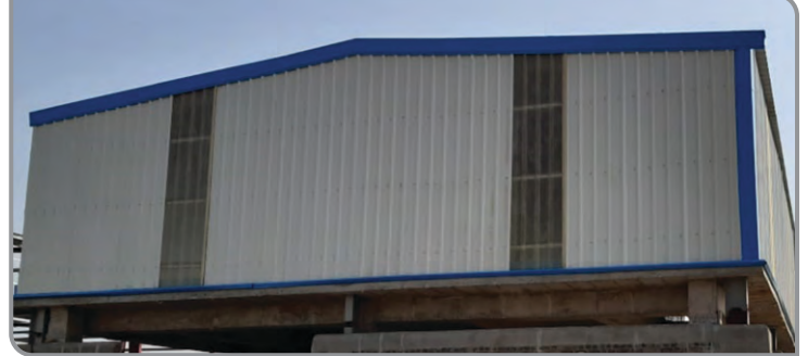
Ghani Ceramics | UTILITY BUILDING POWER HOUSE 22,000 Sft
