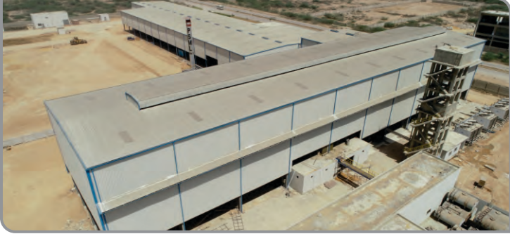
Platinum Steel | Steel Melting Shed 43,143 Sft
